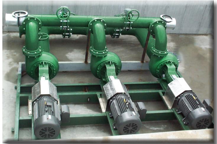
GreenLine 10X8X14 Flush pumps for 24,000 cow dairy with back-up pump.
